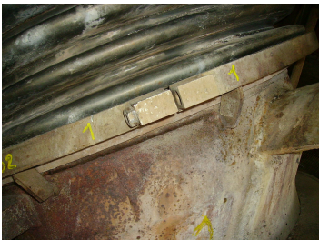
The first reinforcing must be not removed
